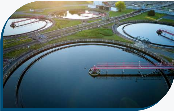
Sewage / Water Treatment Plants
